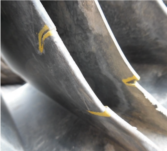
Spoke Edge Cracks
